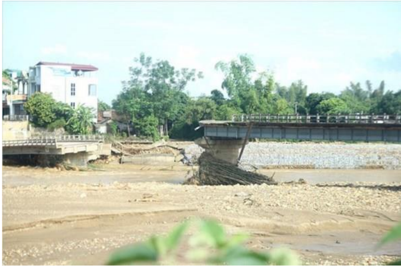
Ngoi Thia Bridge collapsed in Vietnam due to flooding, Dec 2017
